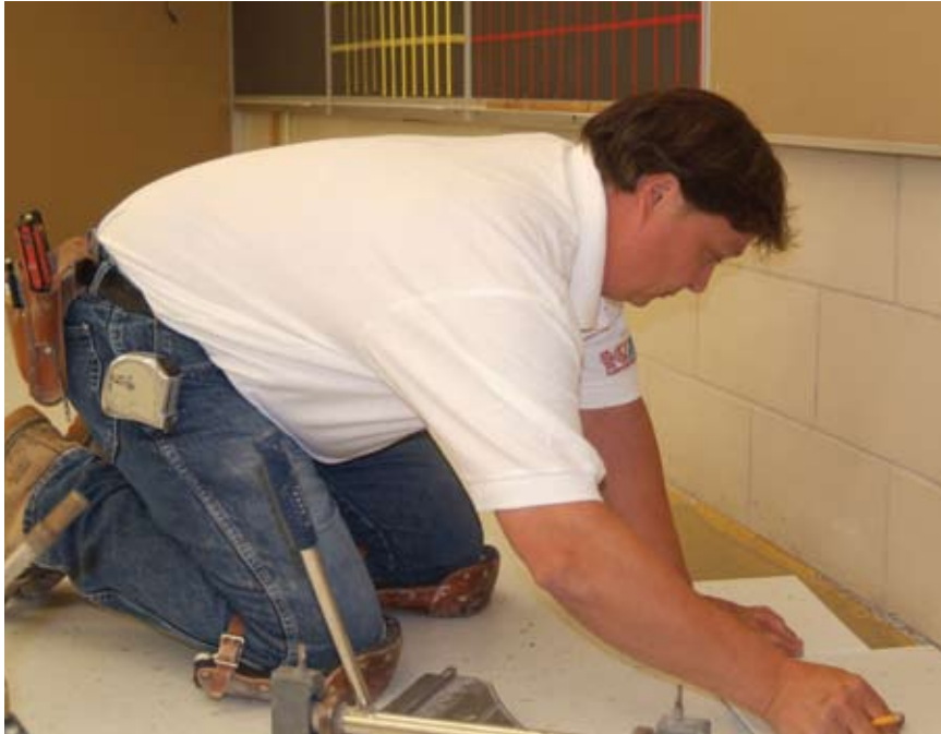
INSTALL professional installing linoleum tiles
