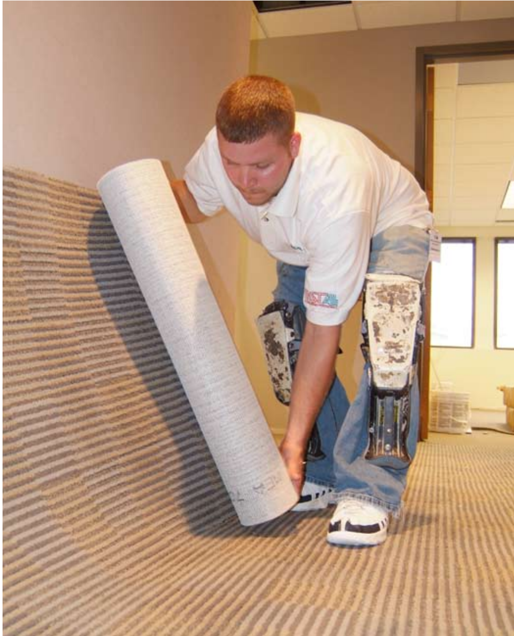
INSTALL professional laying down carpet
